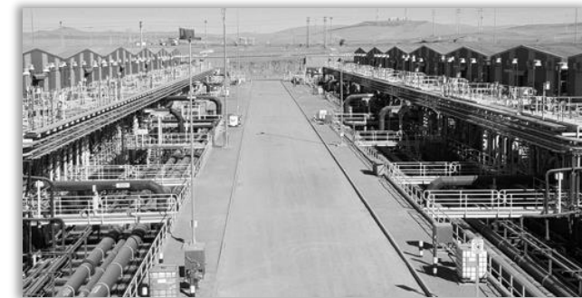
Copper SX Plant - Chile
