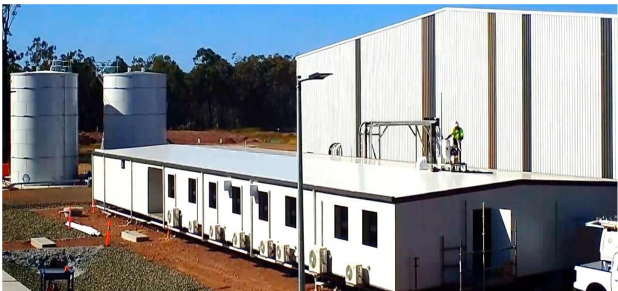
Main administration and laboratory building which was installed in August 2022
