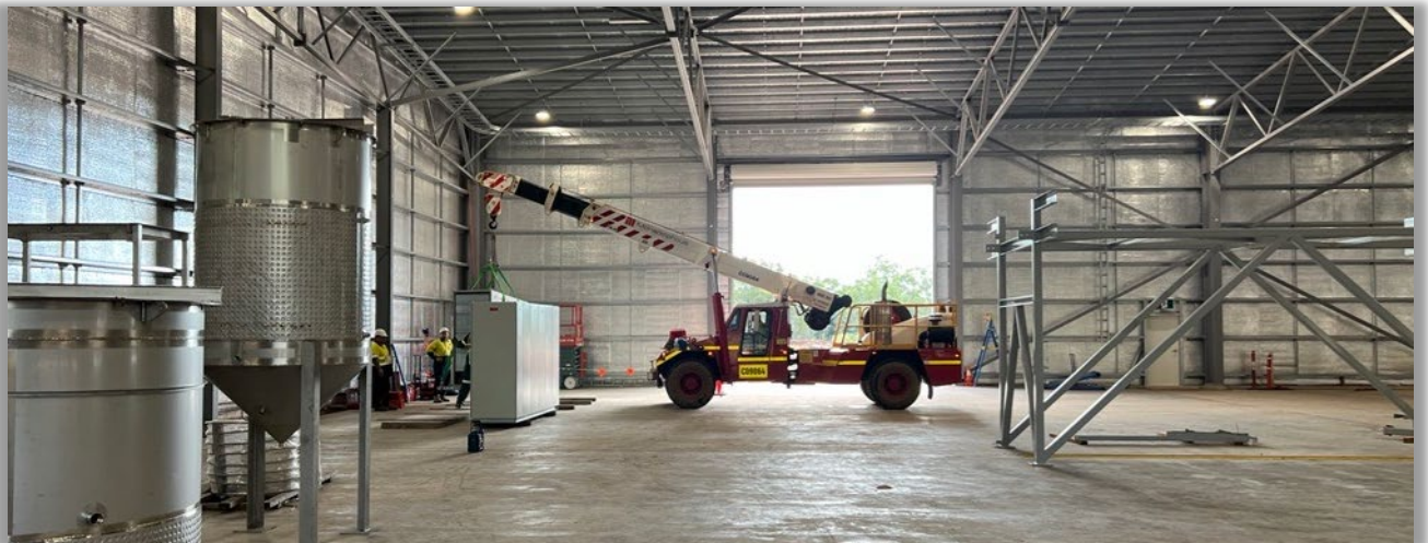
Interior lighting installed and energised with process equipment deliveries continuing
