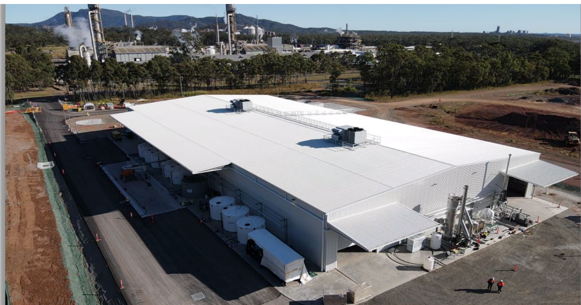
Stage 1 PPF building at lockup stage
