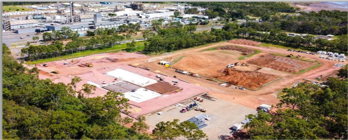
Stage 1 PPF - preliminary earthworks
