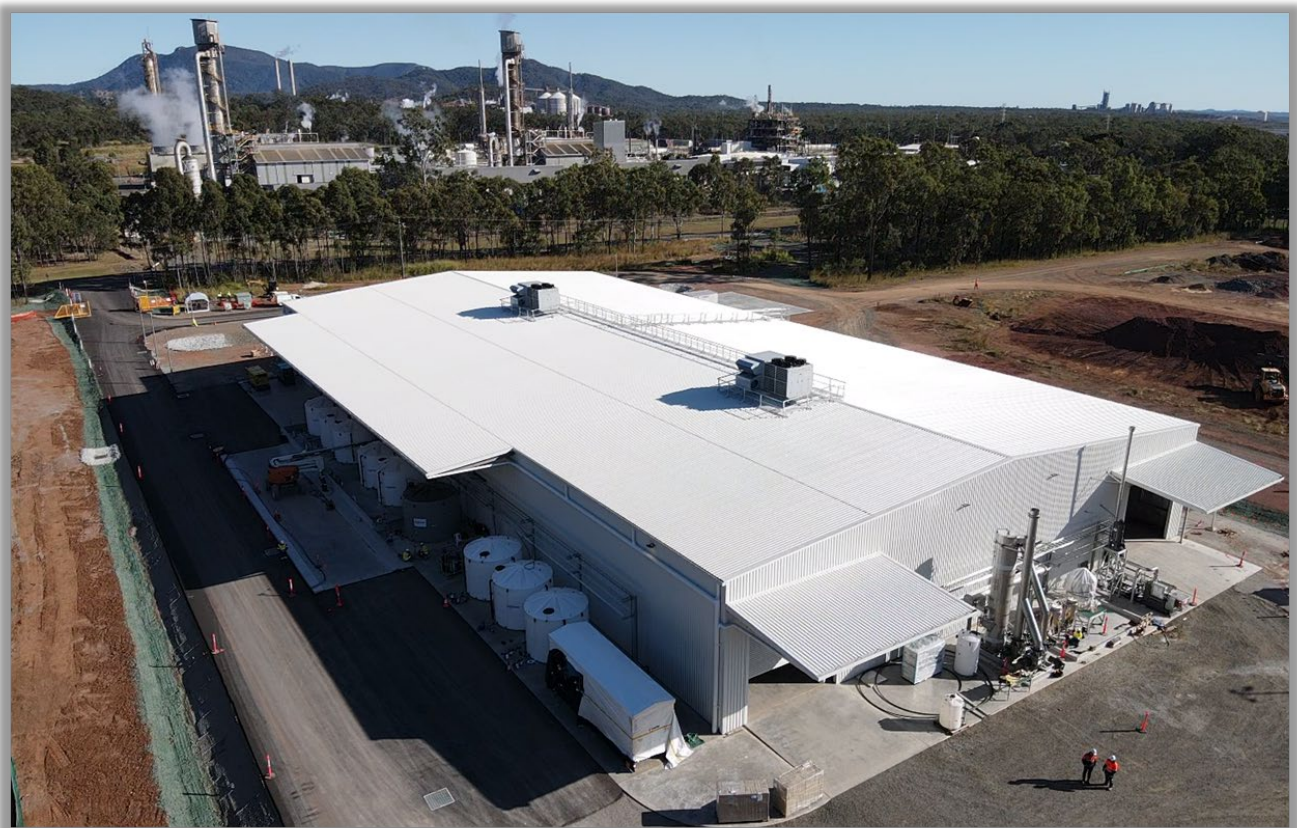
Stage 1 PPF building at lockup stage
