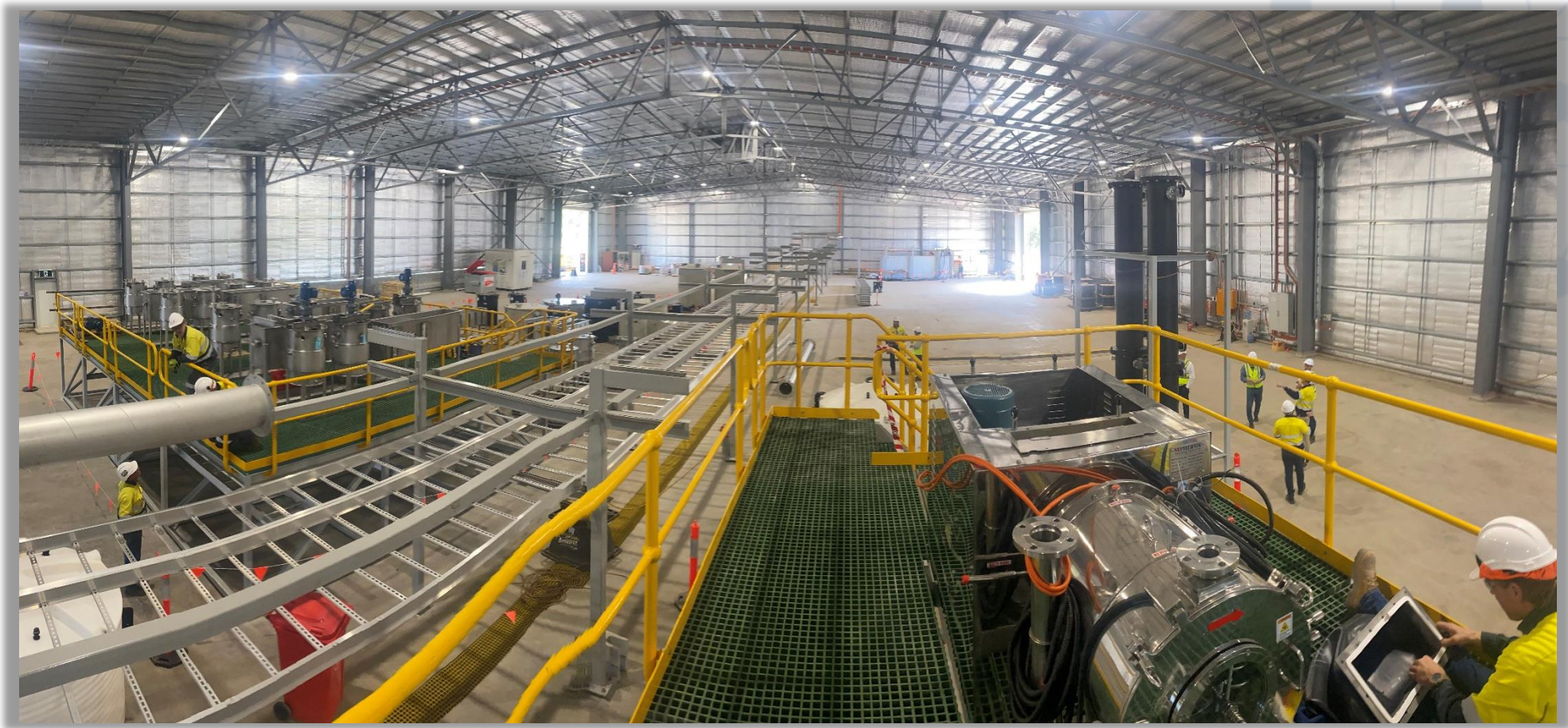
Installation of solvent extraction (SX) circuits
