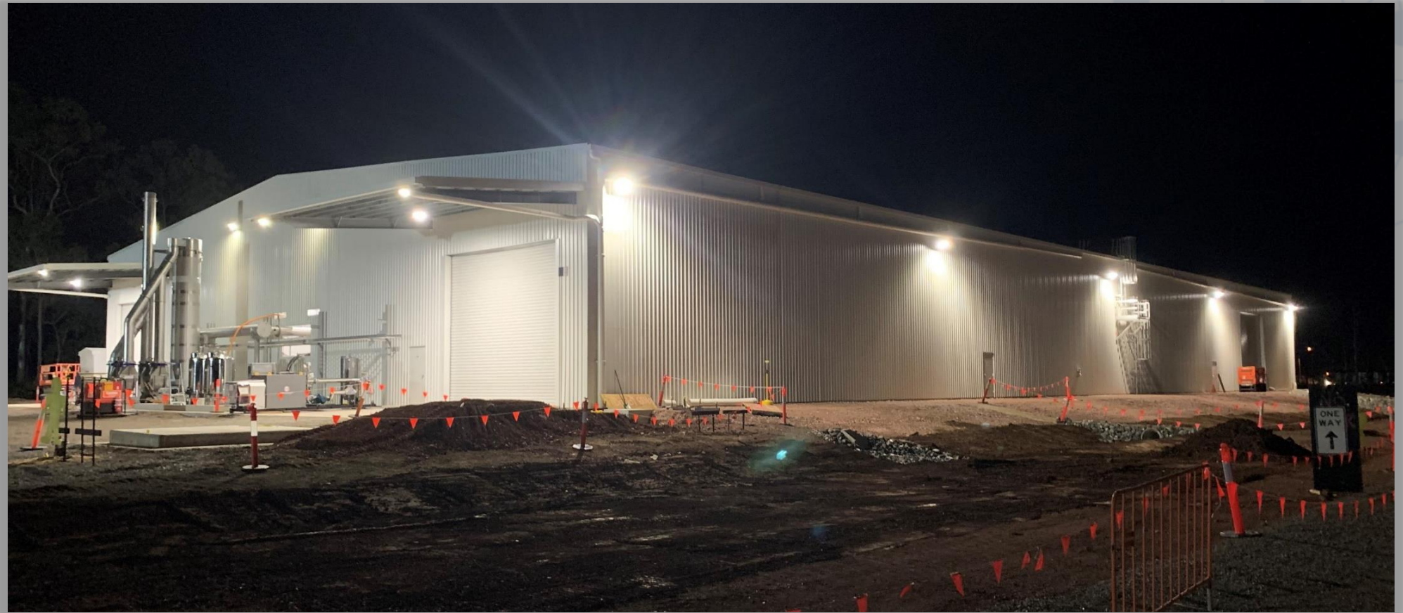
Stage 1 PPF building at lockup stage
